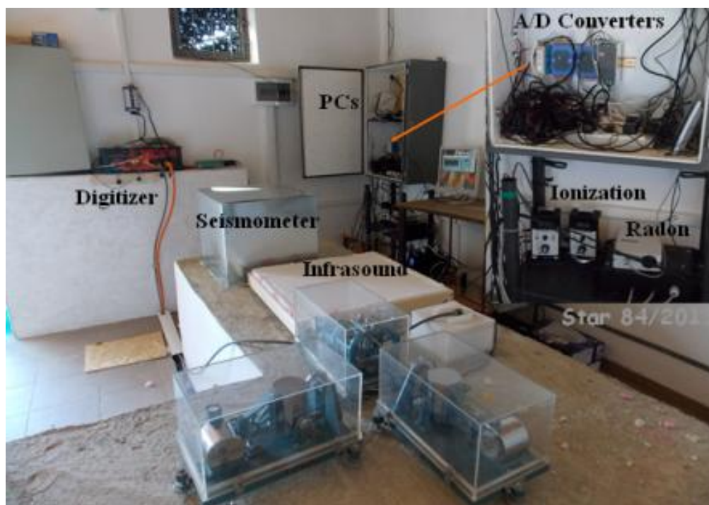
Fig. 2. Multidisciplinary monitoring station in Vrancea
